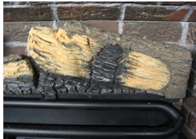
Log "B" installed correctly
