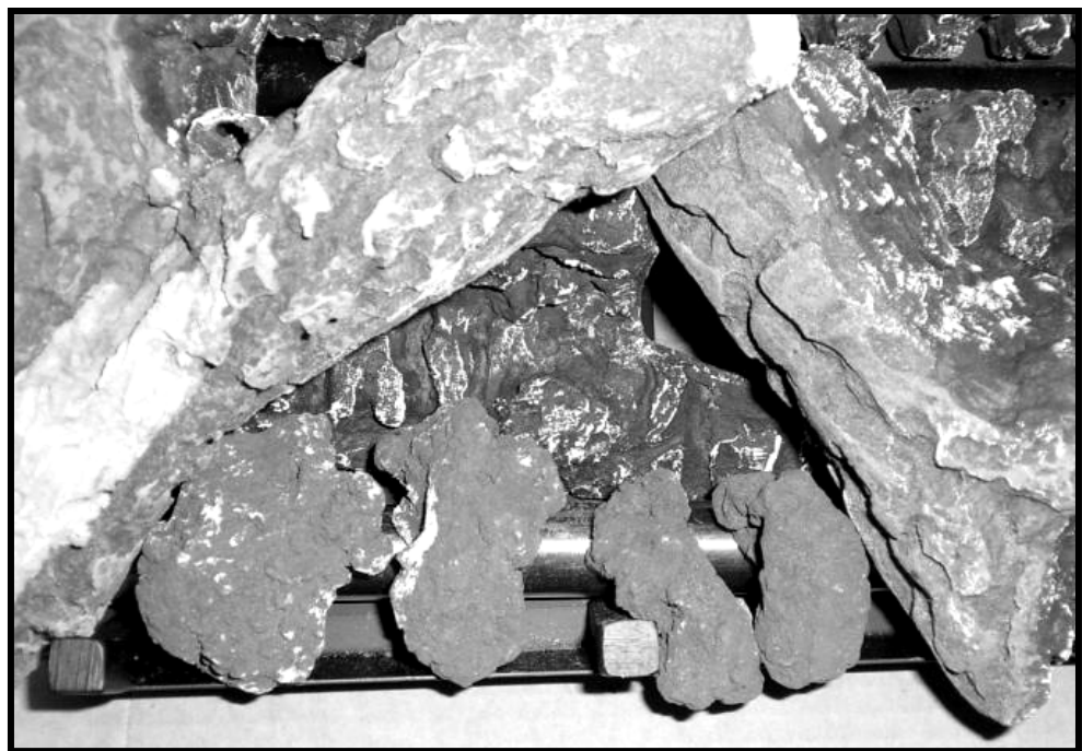
Add Large Chunk Coals behind front burner and on Logs "C" and "D" surfaces. Space Coal Chunks apart at least 1/4" where they touch the Front Burner to allow upward flow paths for Front Burner Flames.
