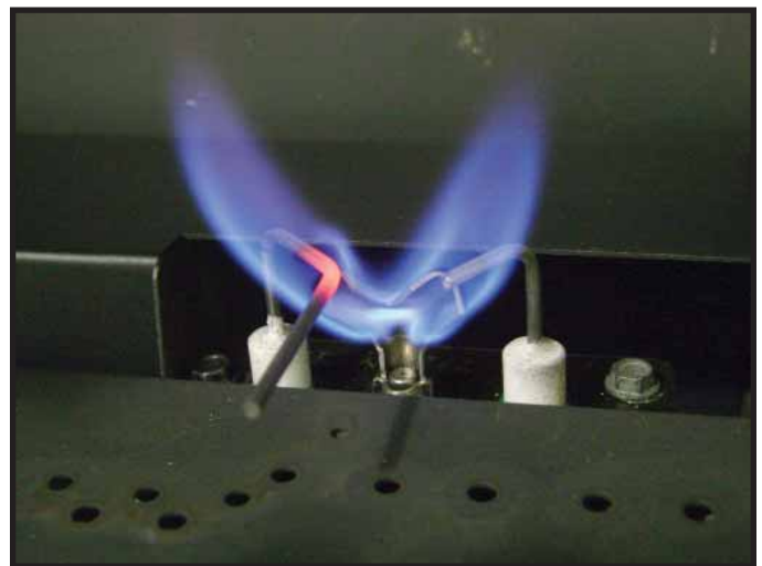
Figure 3.2 IPI Pilot Flame Patterns
