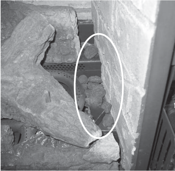
Right side of Burner
